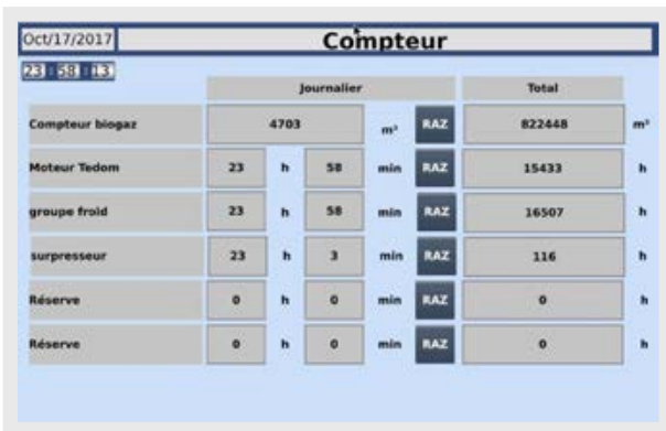
A counter menu that displays values for production volume, engine runtime, compressor runtime, etc.
